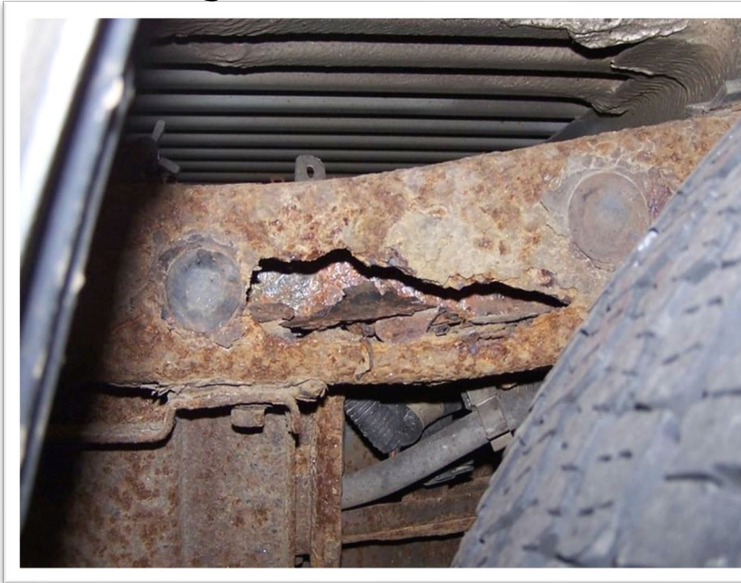
Frame rot and structural integrity
